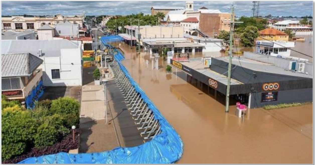
Figure 29 - Inflatable temporary flood barrier
