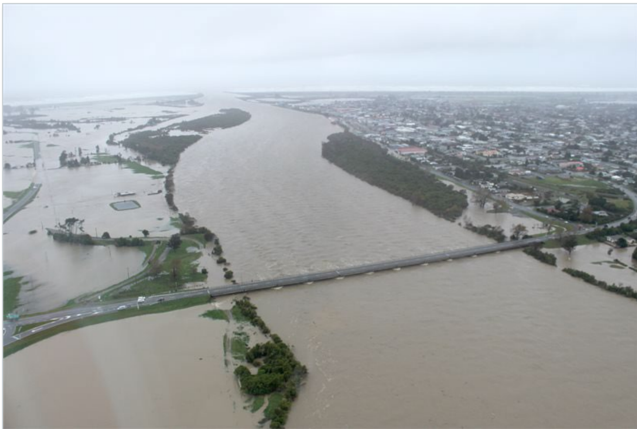
Figure 8 - Flood waters at the Buller Bridge, July 2021
