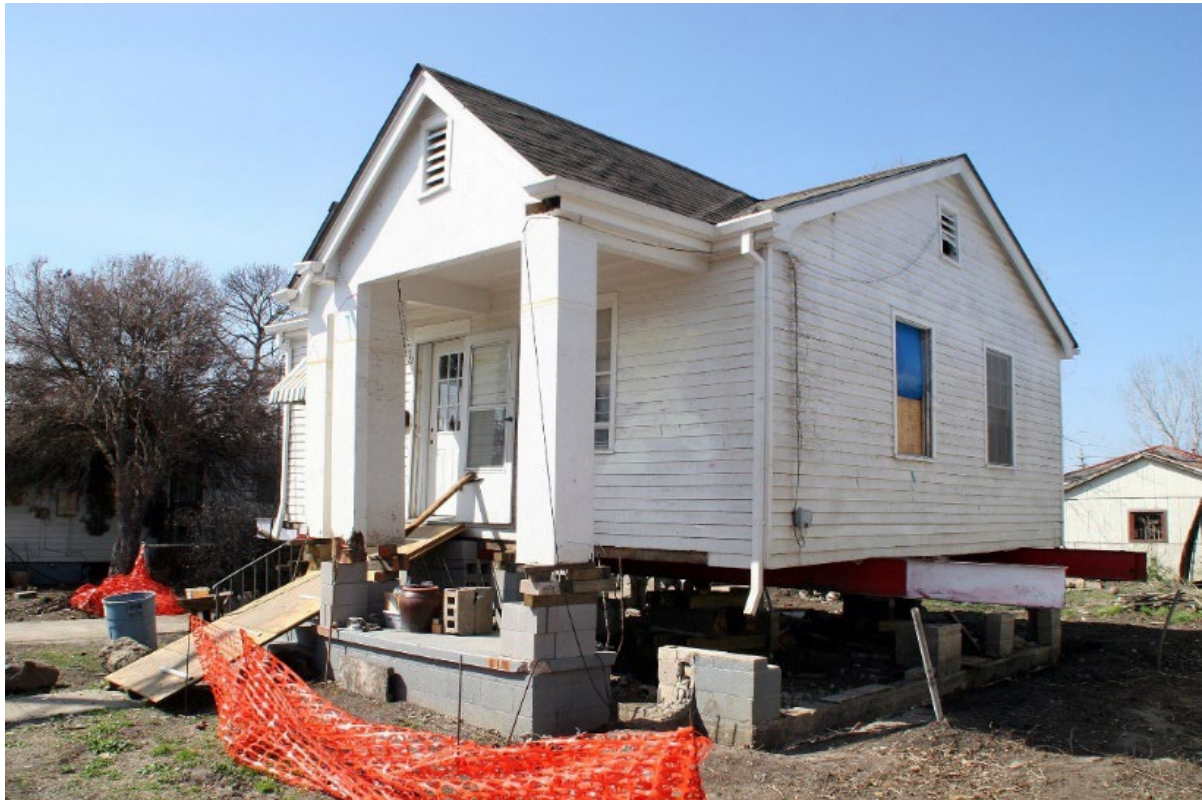
Figure 25 House being raised in New Orleans
