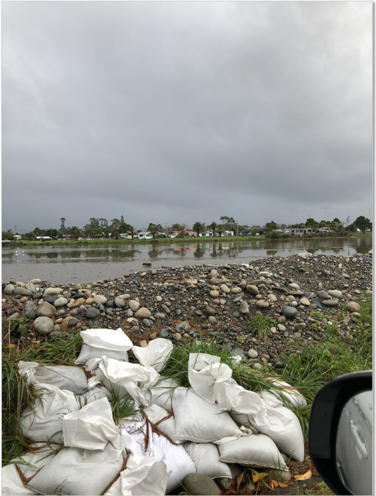
Figure 15 – Temporary stopbank at Snodgrass Road
